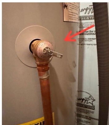
Temperature Pressure Relief (TPR) valve
