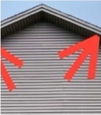
Roof (Drip Edge) Flashing
