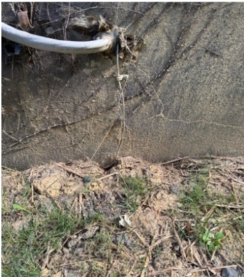
Ground Electrode Con- ductor (GEC)
