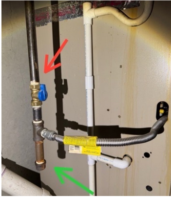
Fuel shut-off (RED) Fuel drip-leg (GREEN)
