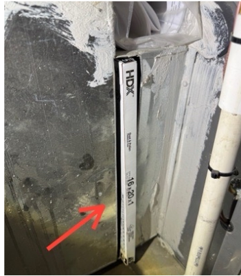
Filter housing and filter
