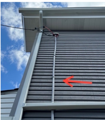
Ground Electrode Con- ductor (GEC)
